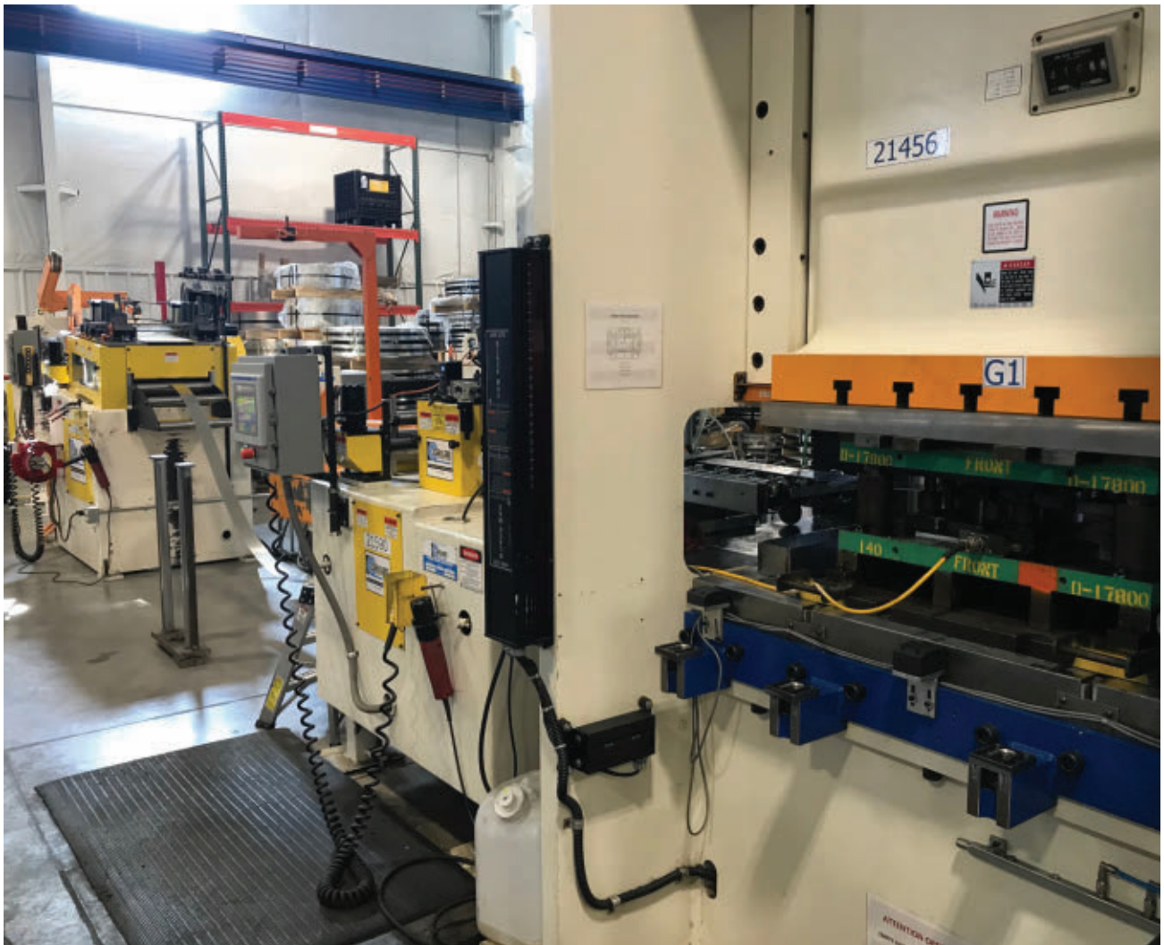
Greenheck Fan Co. installed a Dallas Industries automated feed line for its new servo press to improve changeover time from job to job. Photo courtesy of Greenheck Fan Co.
